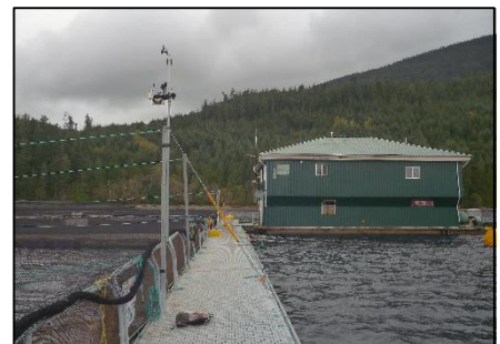
Image 2. Weather station installed at fish farm.
