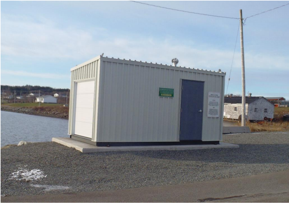
Example of a building specially designed to house used oil tanks, with proper ventilation and in-floor spill containment.
