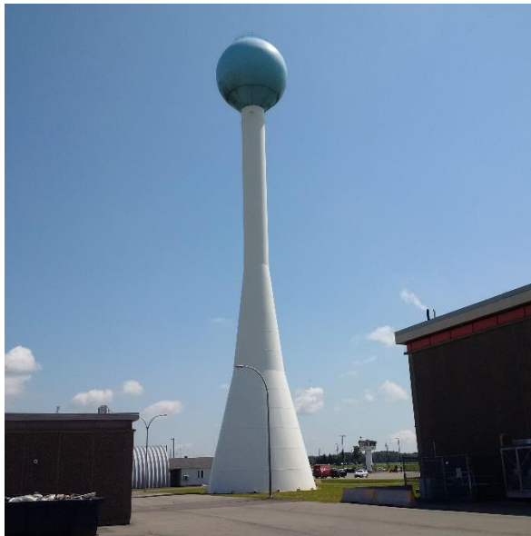
Water Tower, Archambault Complex, QUE
