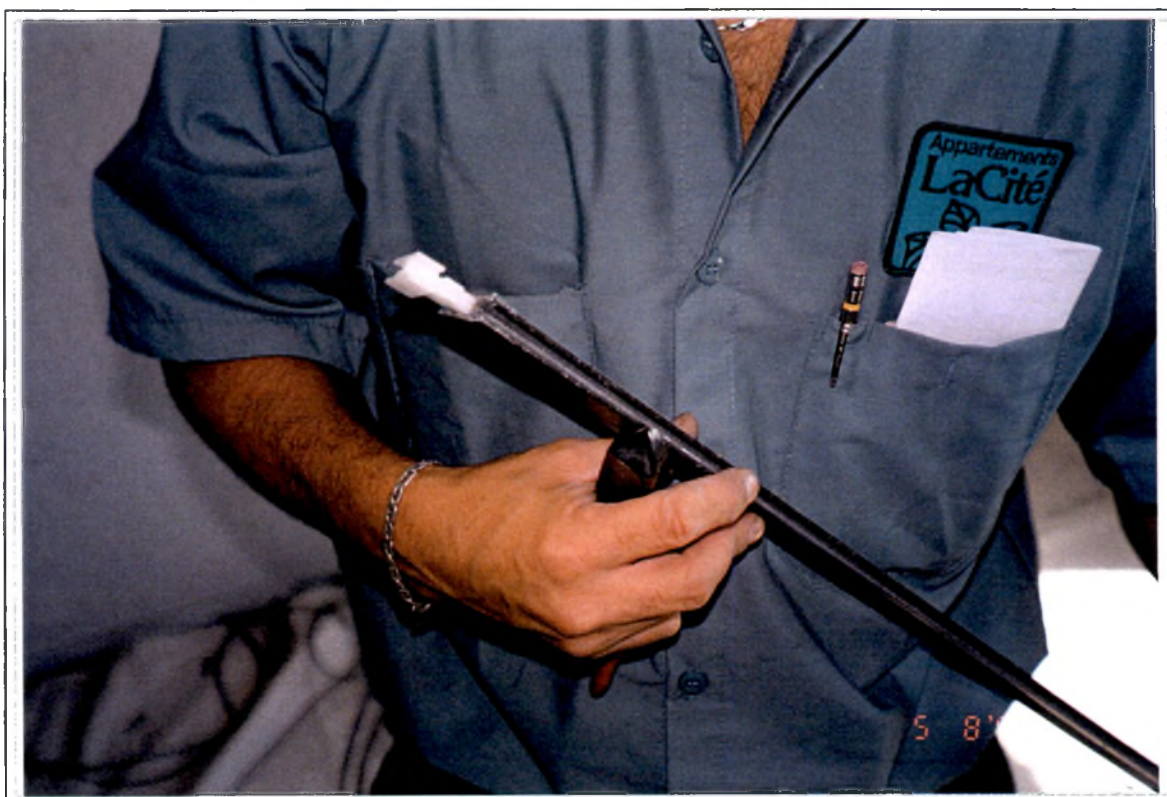
Photos #8: Maintenance worker from the La cite aptmnt complex holding a sash sill with newly installed weatherstripping. Note the plastic glider at the end of the sash sill.
