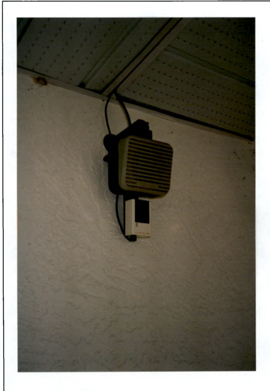
Figure 3 Front Door Camera and Intercom System.
