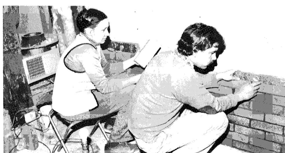
Jack and Sue are laying thermal bricks on the first floor of the addition. Jack said the thermal bricks will help retain daylight heat and release it in the evening.
