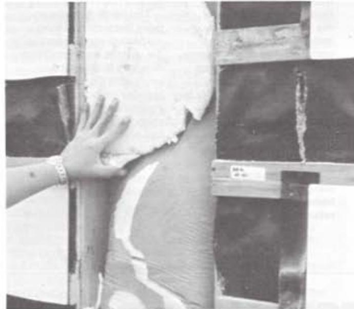
Example of poor application of foam that caused it to shrink.
