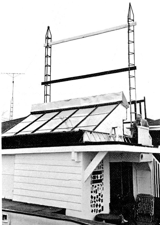
Claude checks the fan for his proposed windmill system. When the windmill system is added to the solar heating unit it will ensure that the Smiths' house is evenly pressurized against draughts.
