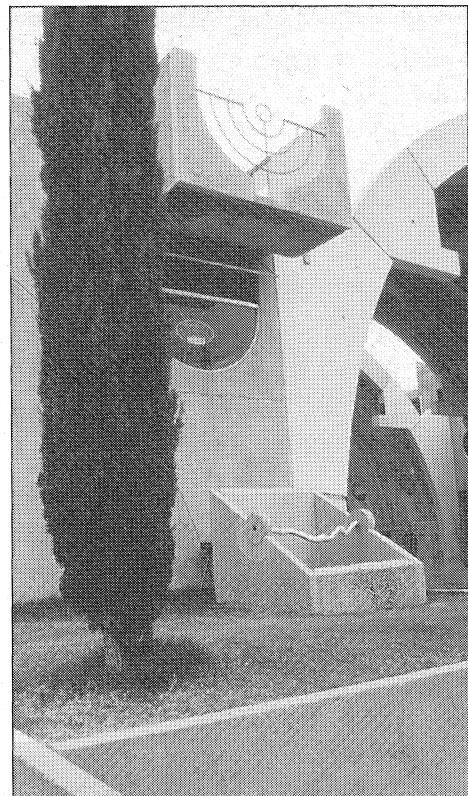
*Rain – infrequent in the desert – runs off the roof into a cistern for later re-use.*
