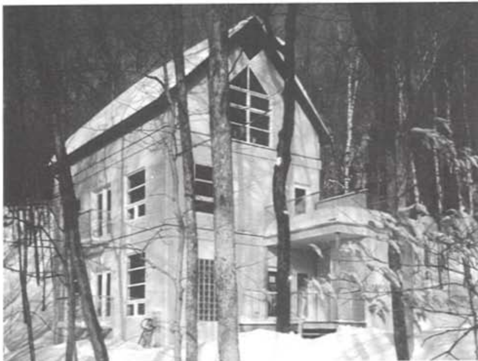
Flex-Housing project in Saint-Nicolas, Quebec.
