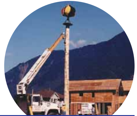
A wind turbine being set up in the centre of the spiritual healing garden.
