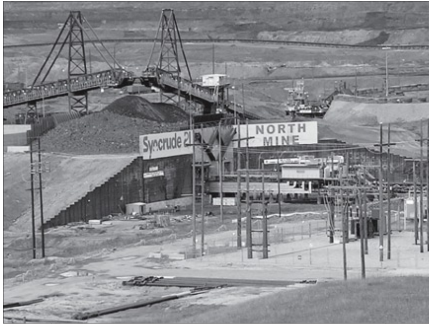
Syncrude facilities in Fort McMurray, Alberta Installations de Syncrude à Fort McMurray, en Alberta
