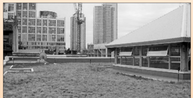
The green roof at the Mountain Equipment Co-op store in Toronto.
