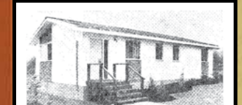
A new approach to housing for families of low income. This three-bedroom modular home features new materials and new construction techniques. A vinyl and wood panel exterior and vinyl floor.
