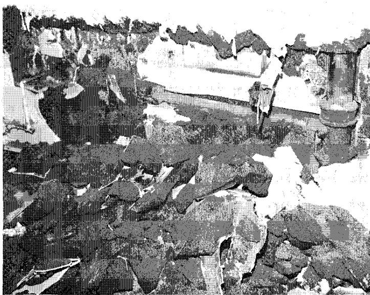
**ON THE OTHER SIDE** — When workmen picked at the foam glass, it fell away in big chunks and revealed the fixtures on the other side of the wall.
