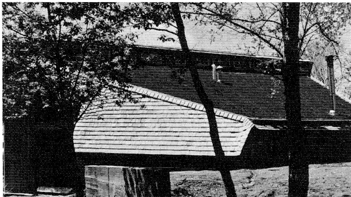
The rear view of the solar house shows the sod roof and the diminished northerly exposure both of which minimize heat loss.
