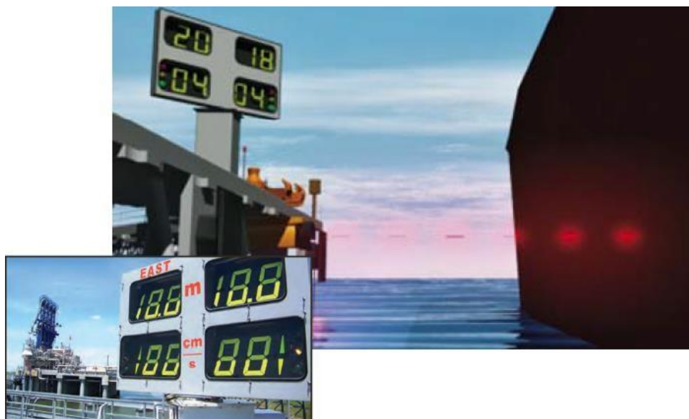
Figure 3.3.2-3 Image of a Jetty Docking Board. Source: Goldboro LNG Presentation to the TRC
