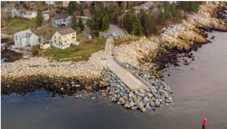
Herring Cove Breakwater – Repaired after being damaged by Hurricane Dorian
