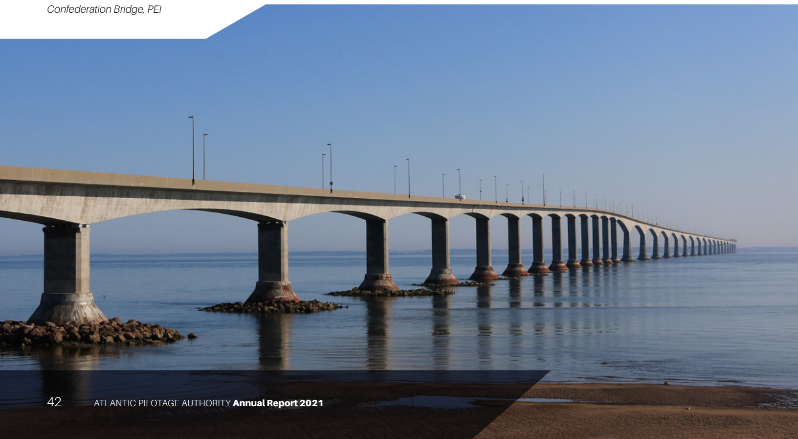
Confederation Bridge, PEI
