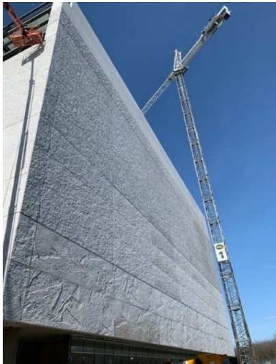
Figure 2: Facade cladding for the new building. The texture is based on the natural geology of the strata below ground level.
