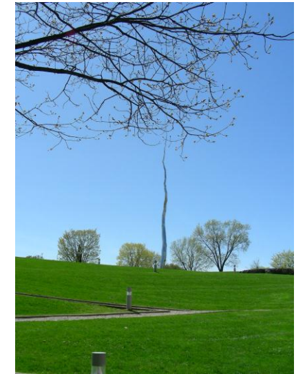
2010: Installation of Roxy Paine's One Hundred Foot Line by the National Gallery of Canada.
