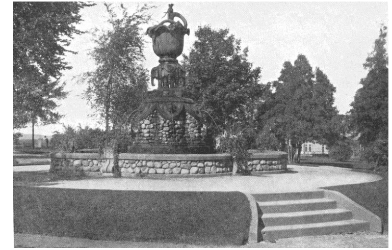
The fountain, made in Osaka, Japan, was offered by Baron Strathcona. It was dismantled and stored in 1925. It was reinstalled and then stored again in 1961 for restoration.
