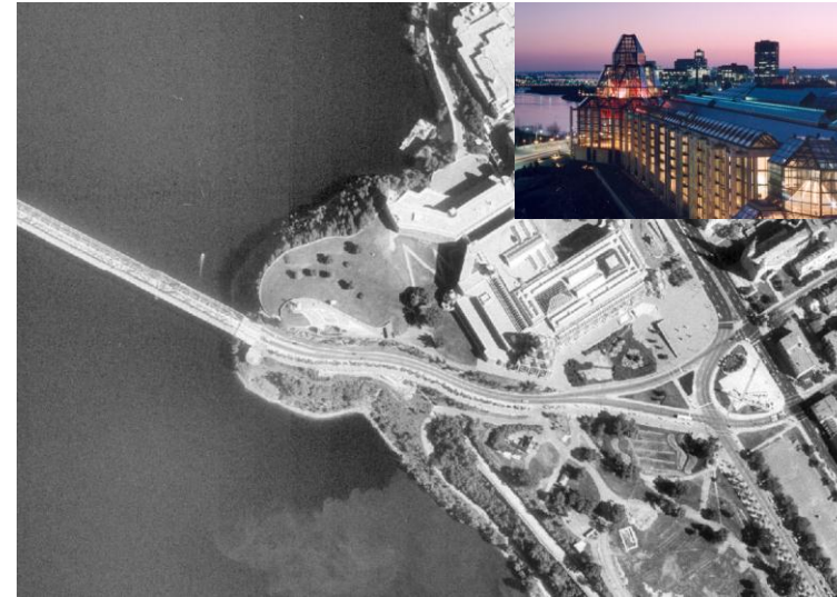
1983-1988: Construction of the National Gallery of Canada, designed by the architect Moshe Safdie.
