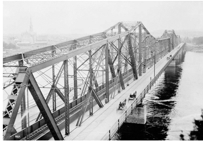
1900: The Dominion Bridge Company built the Royal Alexandra Interprovincial Bridge and the railway splitting Nepean Point and Major's Hill Park.
