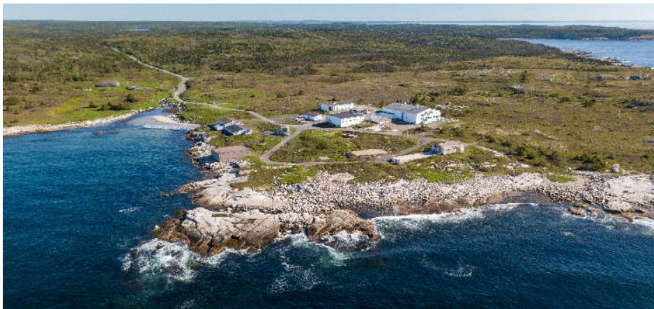
ACRD’s Ketch Harbour facility is a world leading facility in isolation, cultivation, processing and analysis of microalgae and microalgal by-products.
