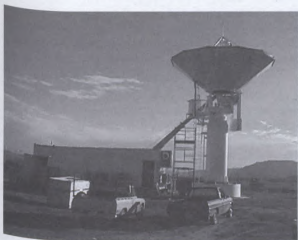
SAN Site under construction
