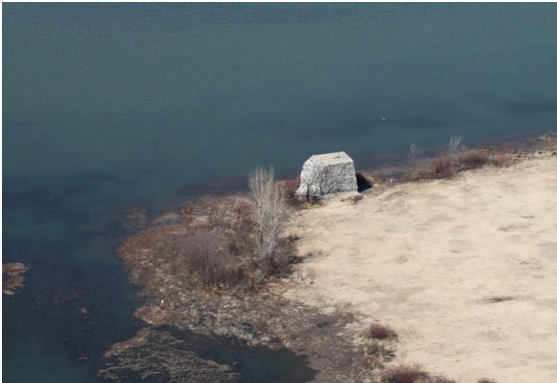
Figure 7: Masonry foundation of a dismantled navigation light, Île de Saint-Chef Photo: Christine Lepage © Environment and Climate Change Canada, CWS
