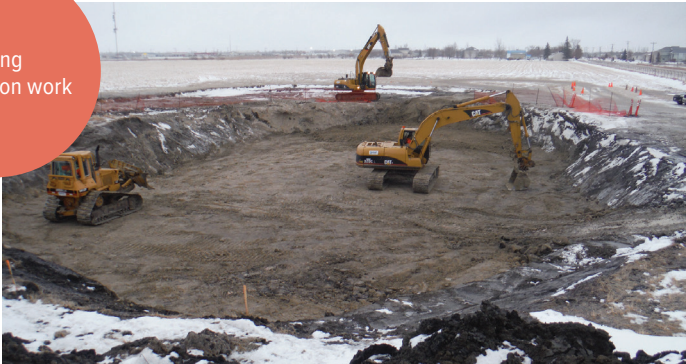
After remediation work
