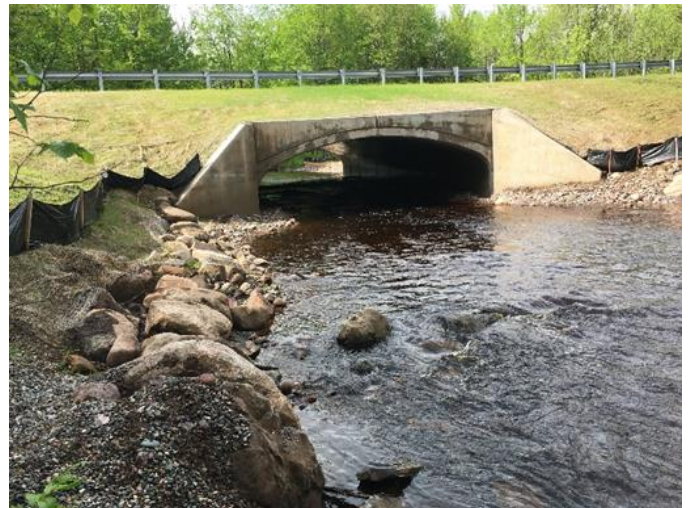
Two Mile Creek culvert replacement – before (top) and after (bottom) restoration. Source: U.S. Forest Service
