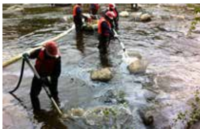
WET TILLING WITH WATER AND AIR INJECTION
