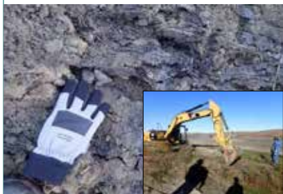
OVERBURDEN REMOVAL TO ACCESS BURIED OIL LAYERS
