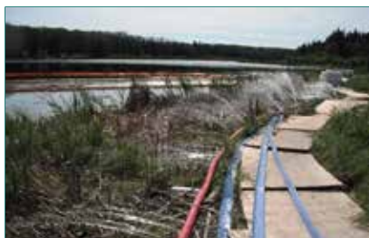
WATER BARRIER (LEFT) AND PHYSICAL BARRIER (RIGHT) TO PROTECT SHORELINE AREA FROM CONTACT WITH OIL
