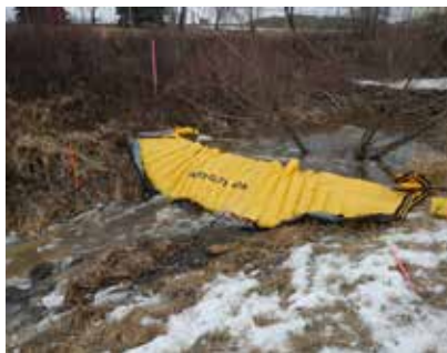
BOOM (LEFT) AND WATER-GATE™ (RIGHT) DEPLOYED ACROSS A SMALL WATERCOURSE
