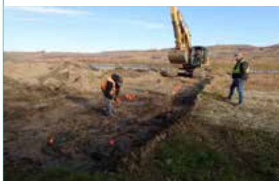
BACKHOE REMOVING UNOILED OVERBURDEN TO REVEAL SUBSURFACE OILING
