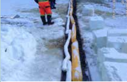
BANK TO BANK ICE SLOT WITH SOLID FLOTATION BOOM/SORBENT BOOM
