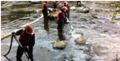
USING WATER JETS TO AGITATE COARSE-MIXED SEDIMENTS
