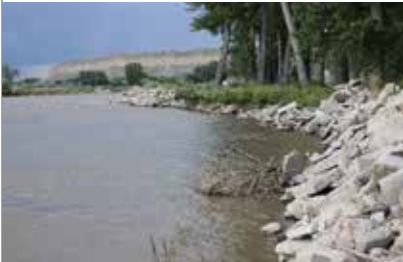
BANK STABILIZATION WITH RIPRAP
