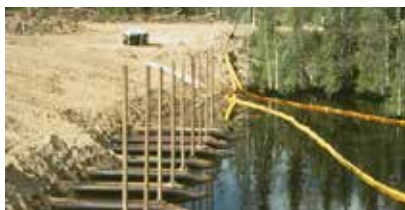
RIVER CONTAINMENT DAM WITH SIPHON PIPES
