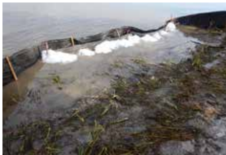
BARRIER FENCE WITH SORBENT USED TO LIMIT REMOBILIZATION OF OIL FROM SHORELINE
