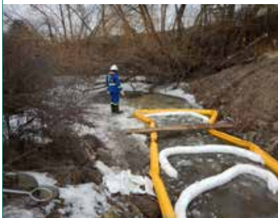
BOOM (LEFT) AND WATER-GATE™ (RIGHT) DEPLOYED ACROSS A SMALL WATERCOURSE
