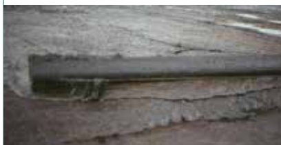
SECTION OF PIPE USED TO SQUEEZE OIL FROM THE FLOATING BOG
