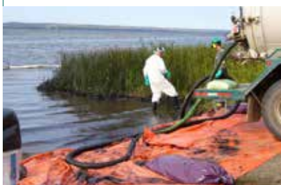
OIL REMOVAL USING VACUUM SYSTEM
