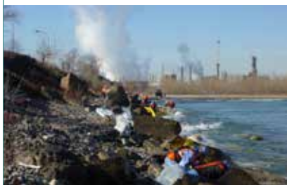
MANUAL REMOVAL OF OIL INTO BAGS FOR COLLECTION
