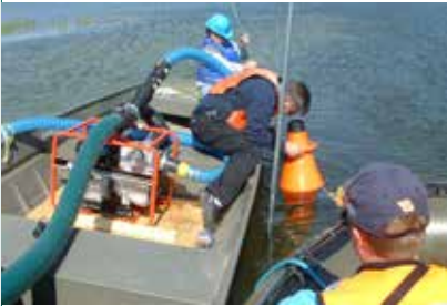
USING A VIEWING TUBE TO DIRECT VACUUMING OF SUNKEN OIL IN NEARSHORE, SHALLOW WATER
