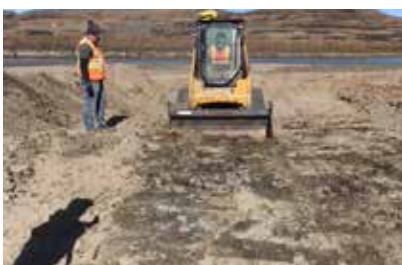
SKID STEER REMOVING OILED SEDIMENTS
