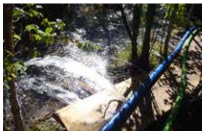
FLOODING SHORELINE WITH PERFORATED HEADER HOSE
