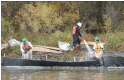
FLUSHING RIVER BANK USING AMBIENT WATER
