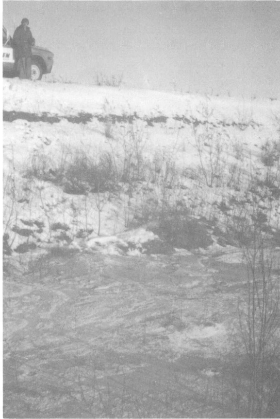
Photo 3 An extensive seepage icing at the end of October, 1973, near the downstream toe of the Inuvik lagoon embankment in an area about 150 m N.W. of the sewer outfall.
