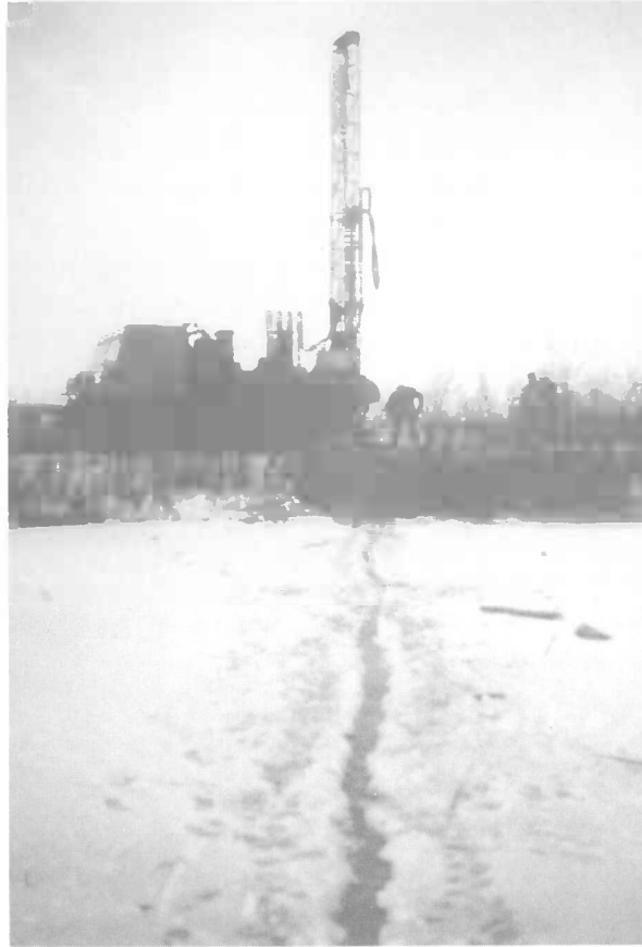
Photo 1 The Nodwell mounted Mayhew rig drilling through the Inuvik embankment. Probe I was lowered through the cut in the ice in the foreground.
