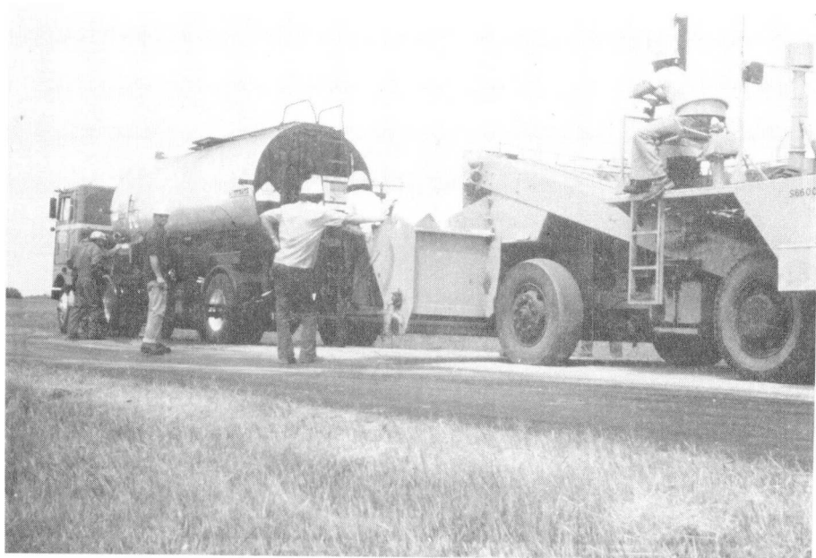
Preparing to Spray R.A.S.
