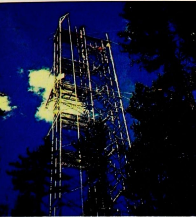
BERMS Instrument Tower
