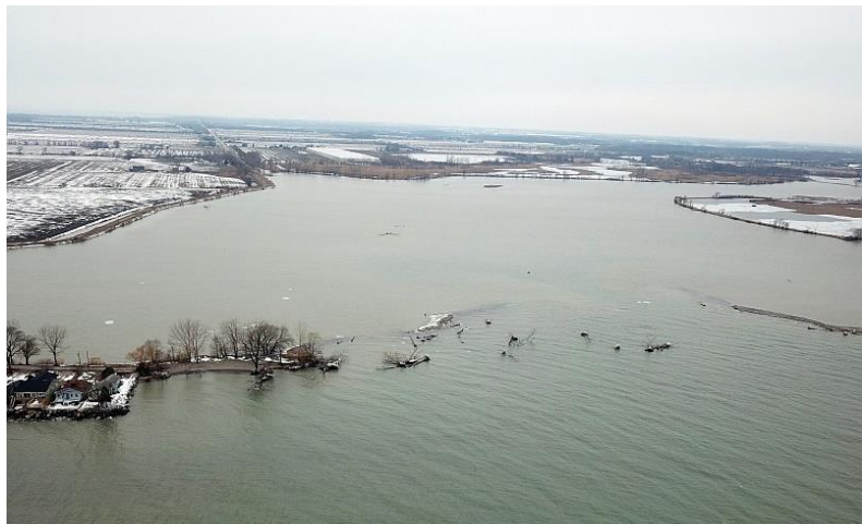
Figure 17. Breach and inundation of the Hillman Marsh barrier-protected wetland (Zuzek, 2020).
