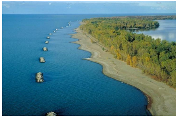
Figure 21. Presque Isle Park barriers.
