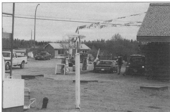
Thanks to EC, fuel storage tanks at this Saskatchewan gas station no longer pose an environmental threat.
