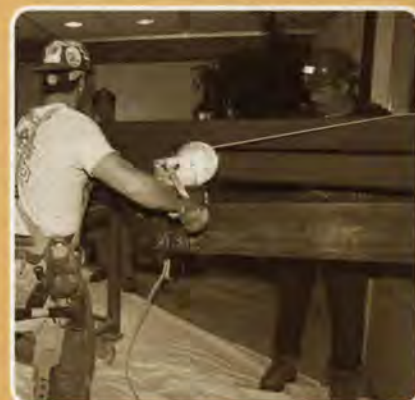
Bringing the beam in through the Minister's window.
