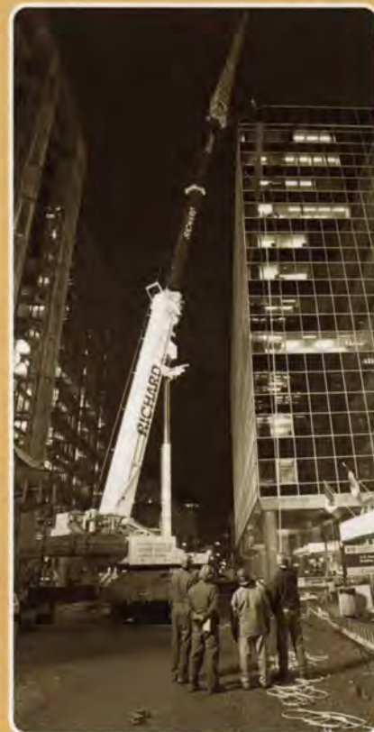
Adding steel-reinforcing beams for the ICDC.
