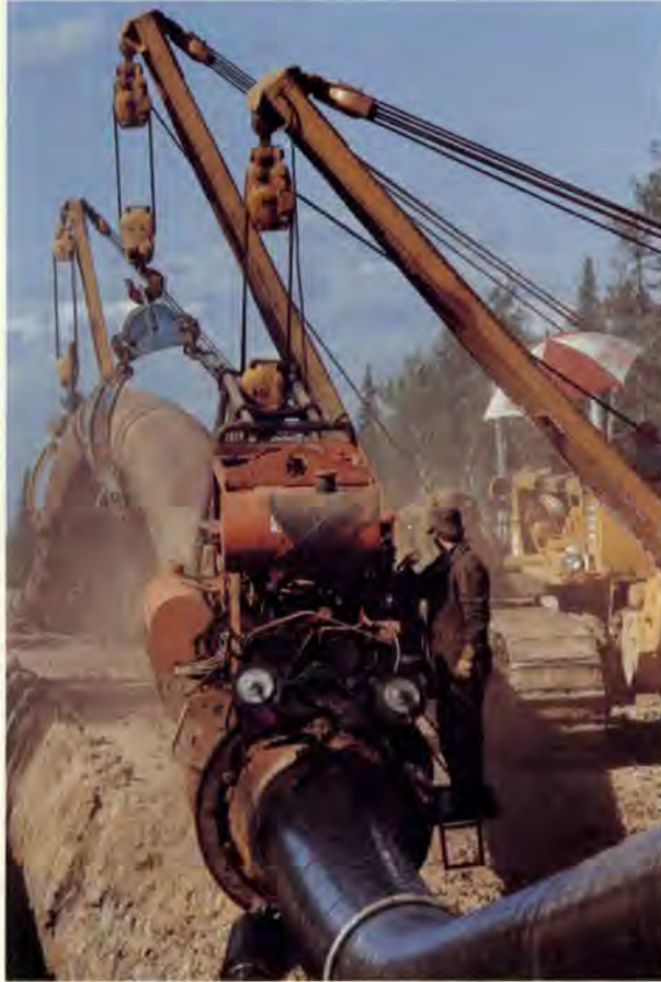
Coating and wrapping a large diameter pipeline
