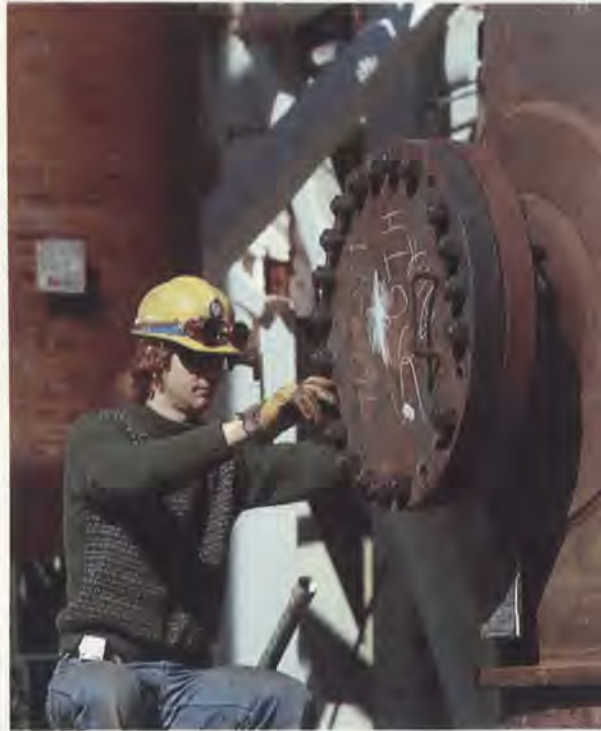
Installing a pressure vessel at an oil sands plant
