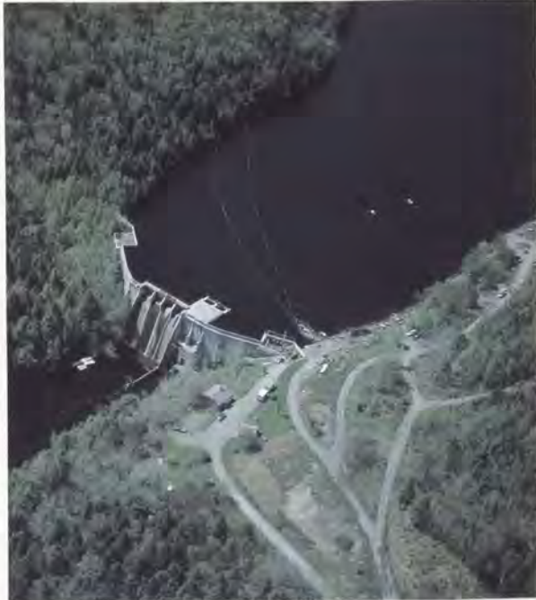
Hydroelectric power dam
