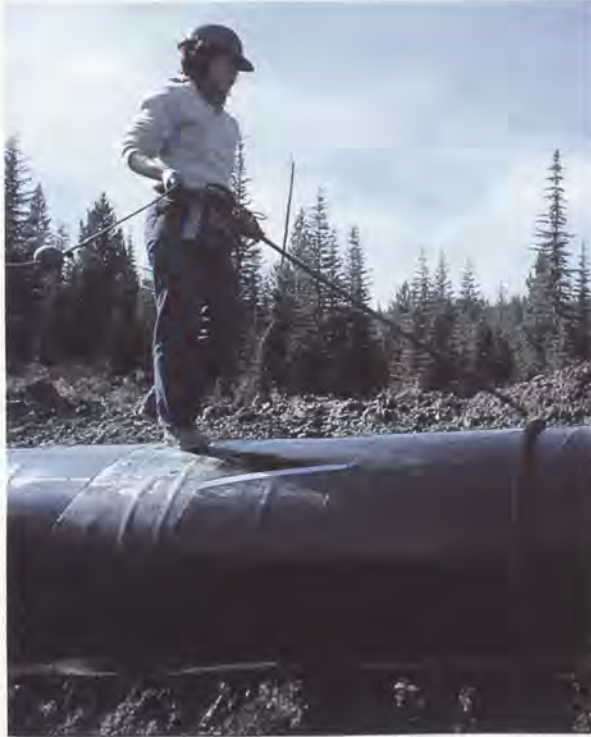
Inspecting pipeline coating
