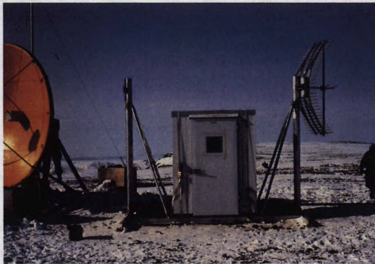
Connecting a satellite terminal to a radio-relay system in the Arctic.
