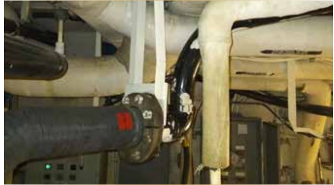
Figure 2. Chilled water supply and return.
