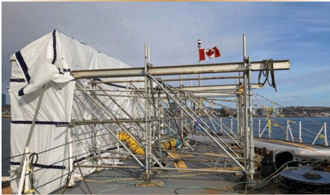
Figure 3. Support structure for the hanging work scaffold.
