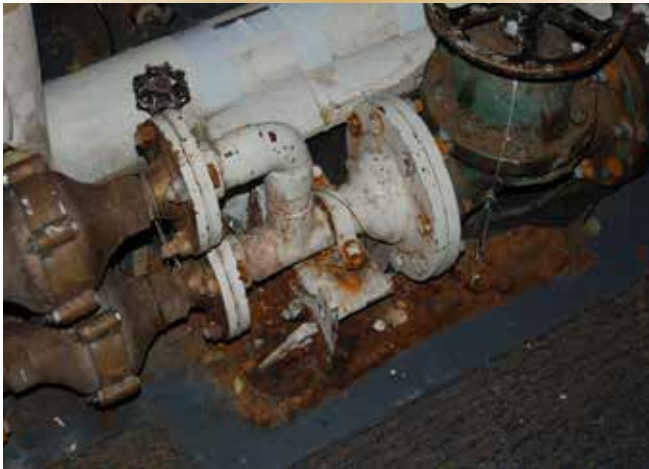
Figure 9. The problem with using dissimilar metals at connection interfaces.
