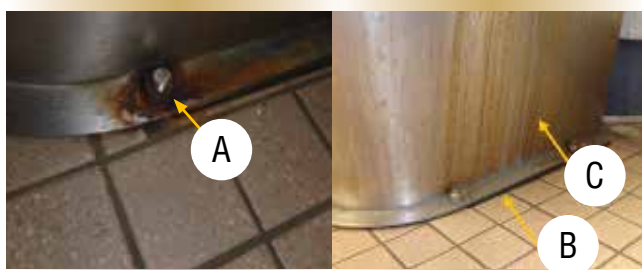
Figure 8. Corrosion on stainless-steel toilets.
