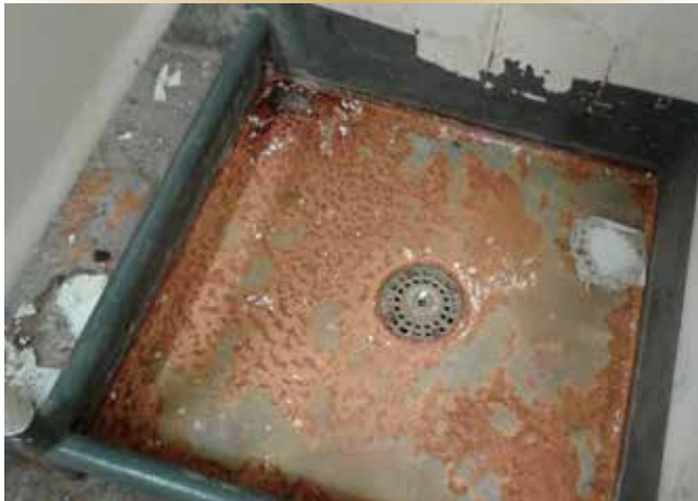
Figure 10. Hidden washplace drain corrosion where the bronze strainer interacts with the mild-steel decking below the tiles.
