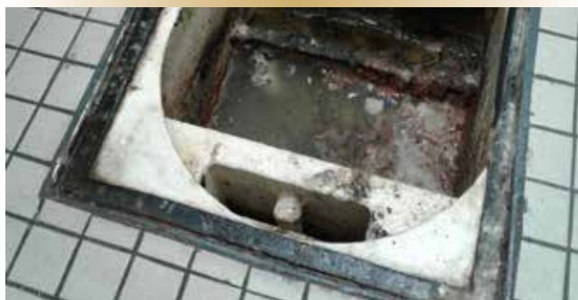
Figure 7. Galley grease trap coating breach and corrosion.
