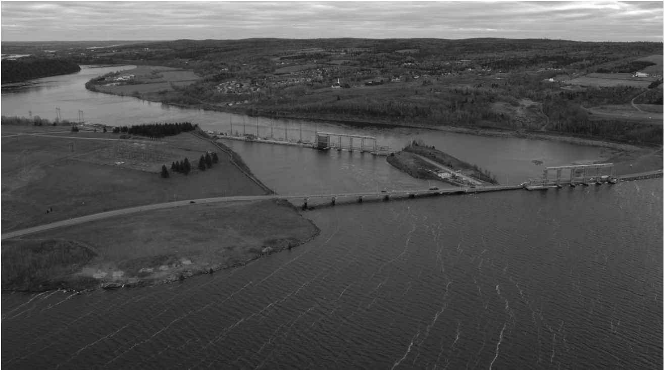
MACTAQUAC DAM — FROM THE WEST (2006)
