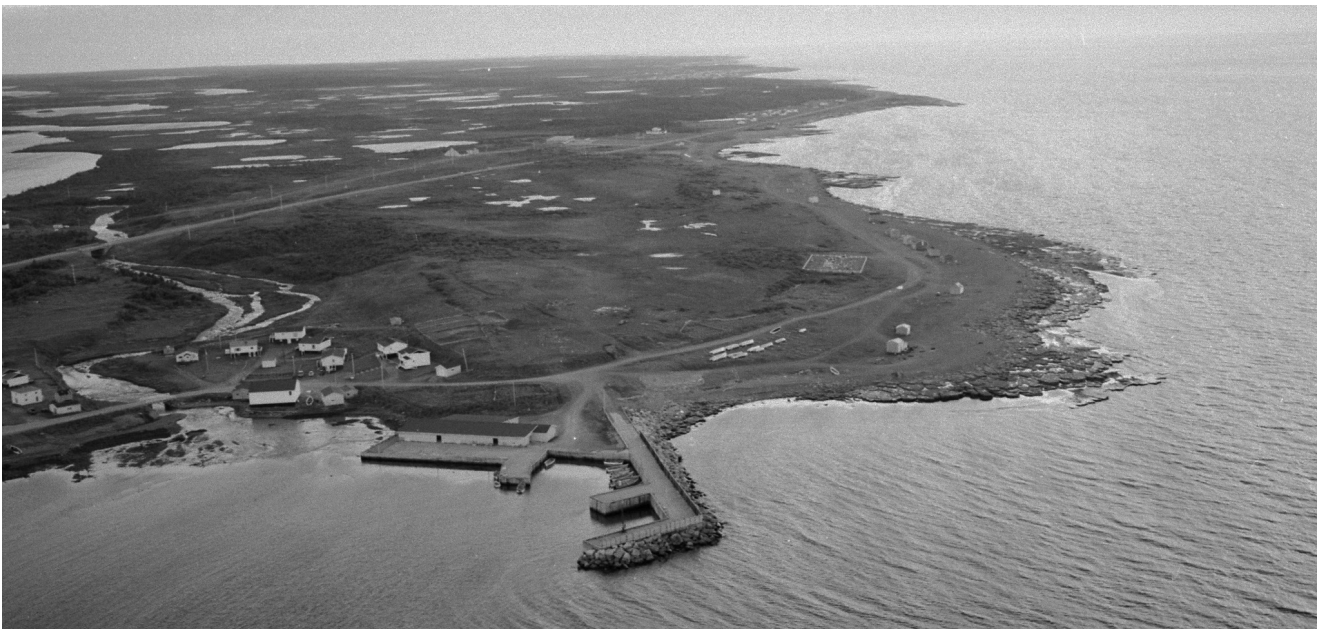
GREEN ISLAND BROOK PUBLIC WHARF (2001)
