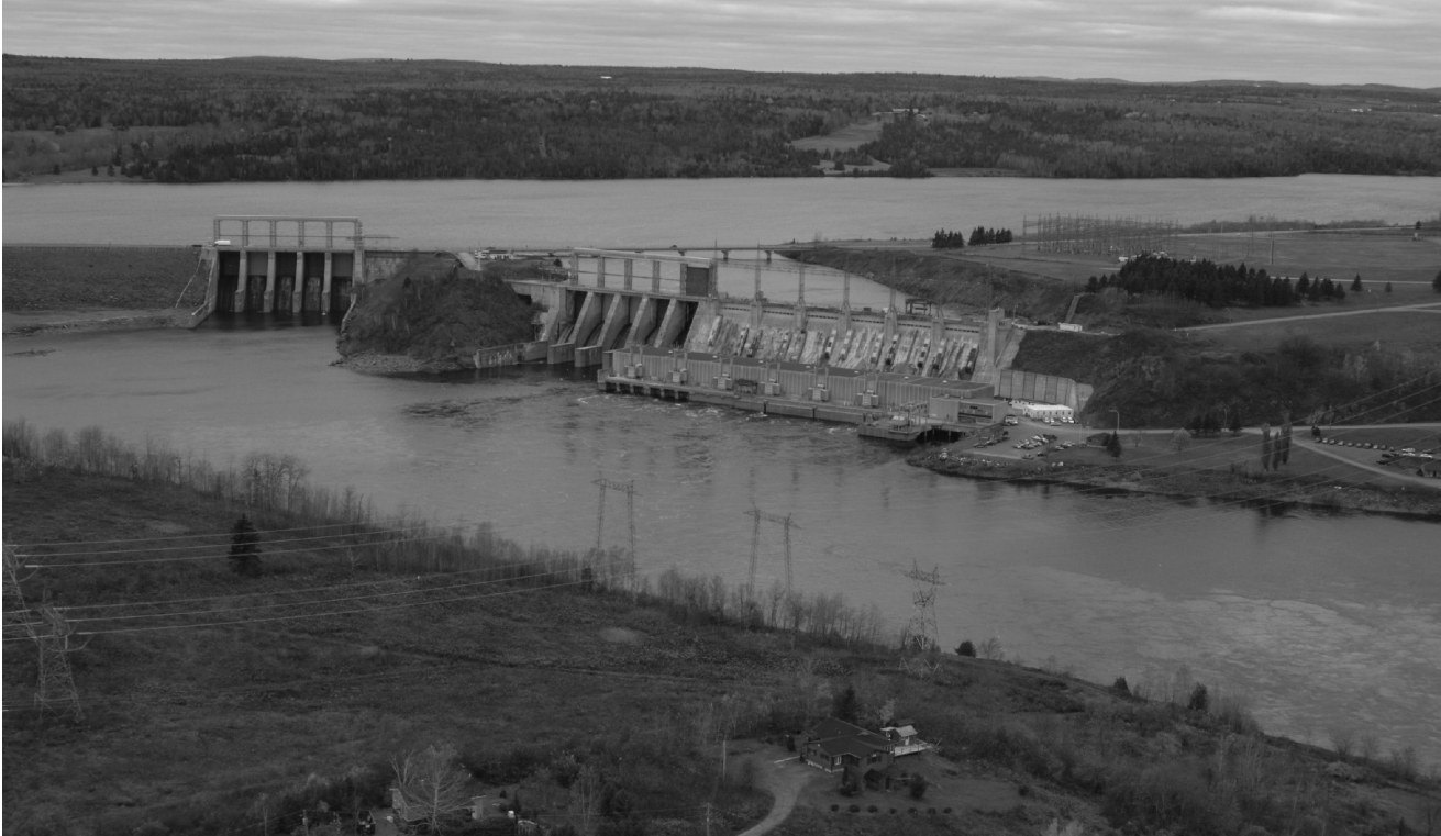
MACTAQUAC DAM — FROM THE EAST (2006)
