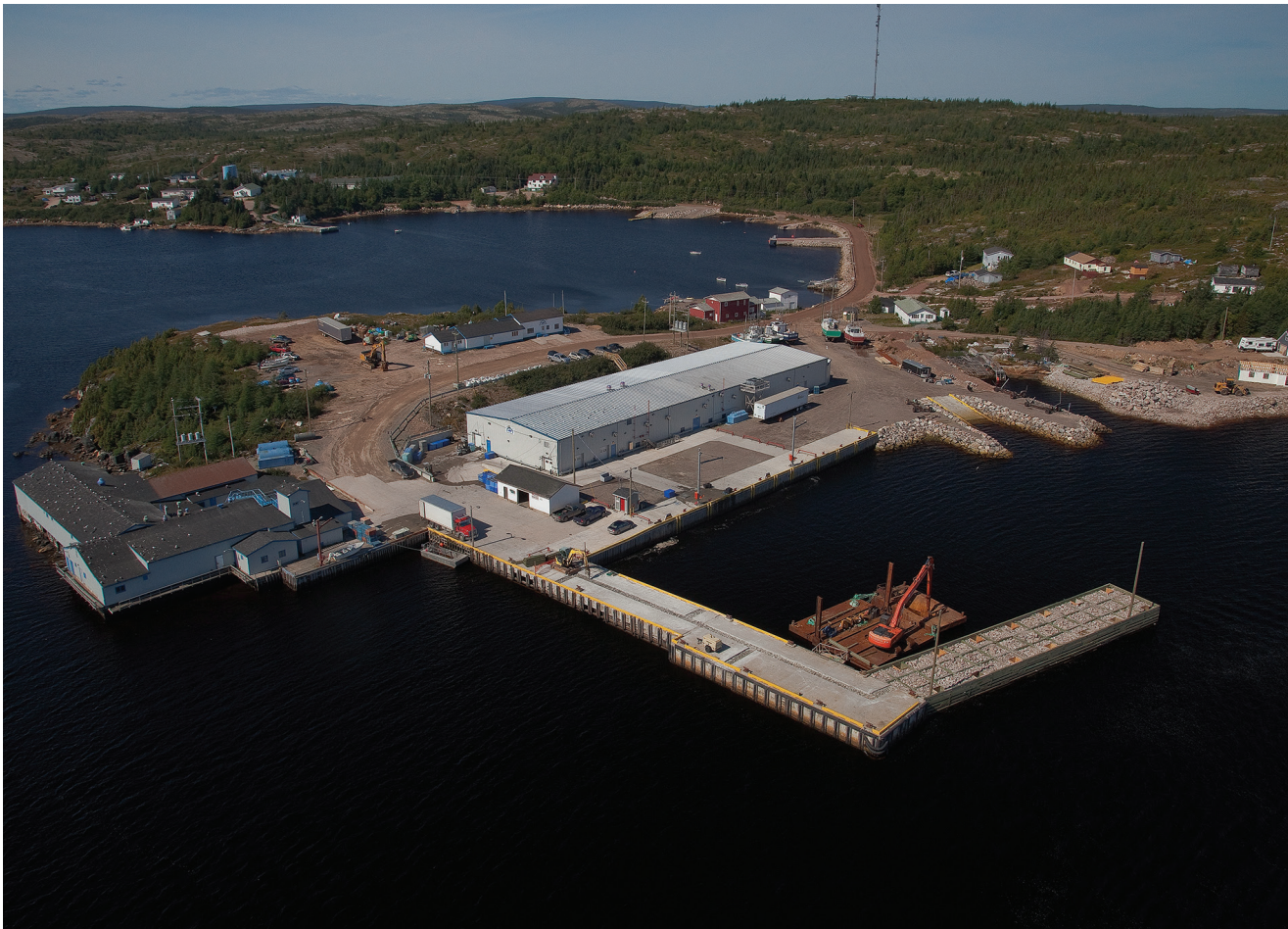
MARY'S HARBOUR PUBLIC WHARF (2015)
