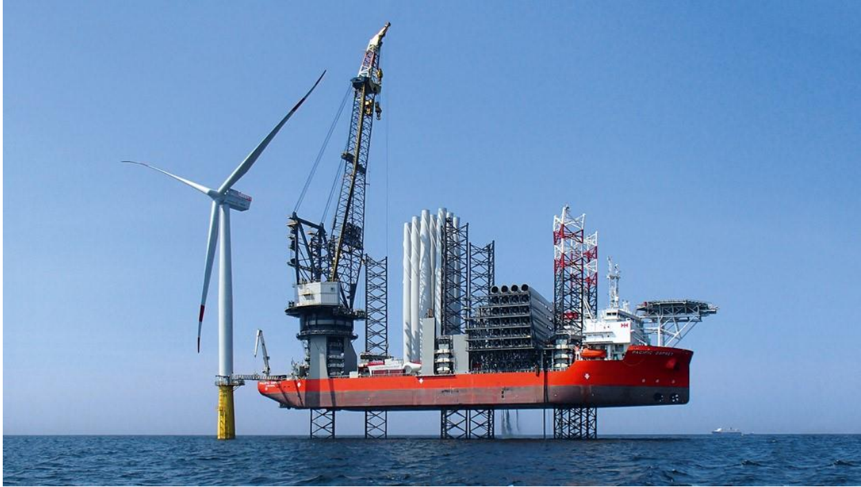
Figure 3.2.1: Offshore wind turbine being erected by a crane from a jack up vessel [35]
