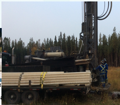
Pipe and screen installation
