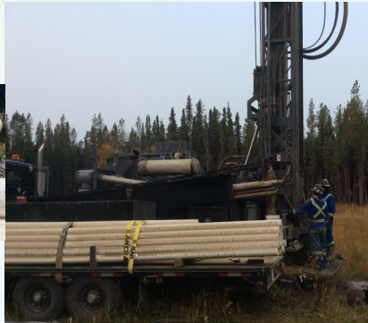
Pipe and screen installation
