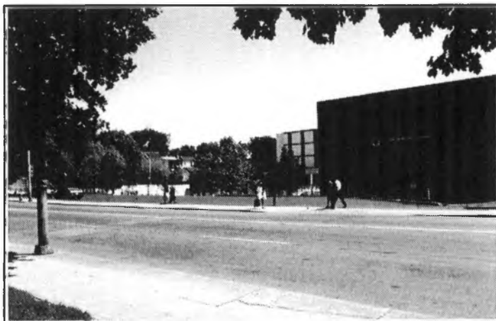
Figure 13: Complicated changes in grade separate the entrance from the street and playground, so that any potential for shared amenities or 'eyes on the street' is lost
