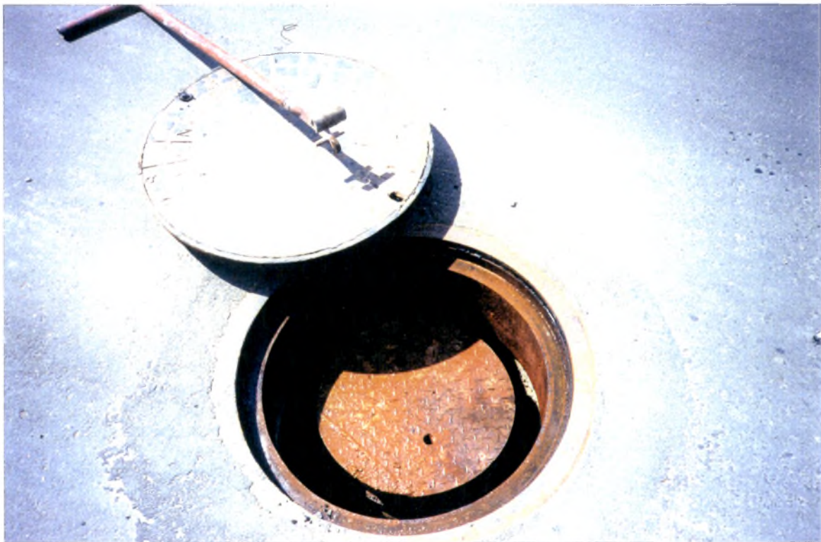
Fig. F: Cover of Alternate Sewer Access Chimney and Precast Concrete Pit
