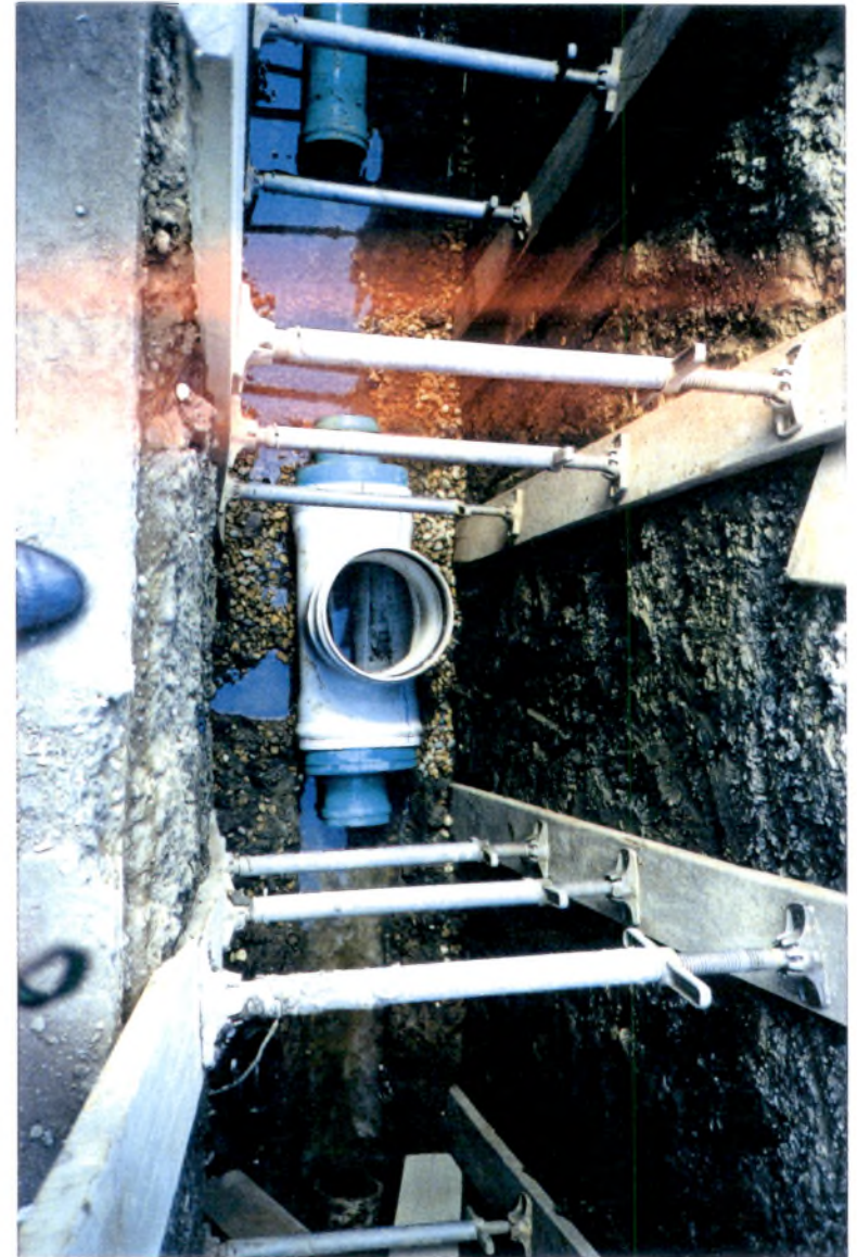
Fig. C: Alternate Sewer Access Base Fittings
