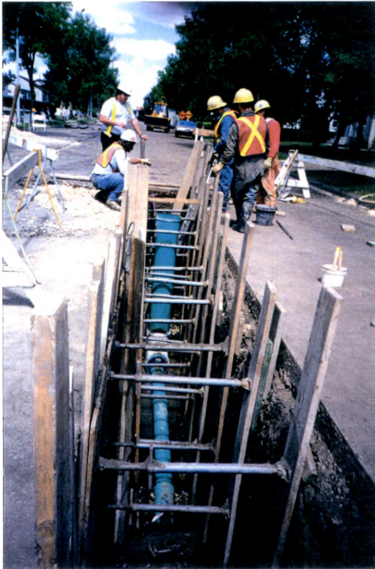
Fig. D: Alternate Sewer Access Connection to Existing Sewer
