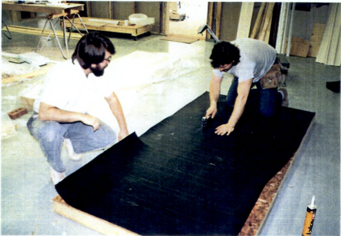
Photo 4 Construction of test panels.
