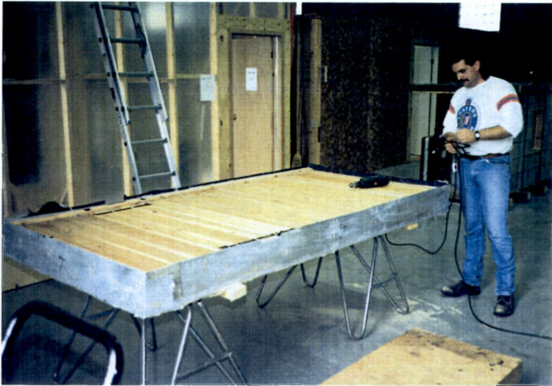
Photo 8 Panel removed for dismantling.
