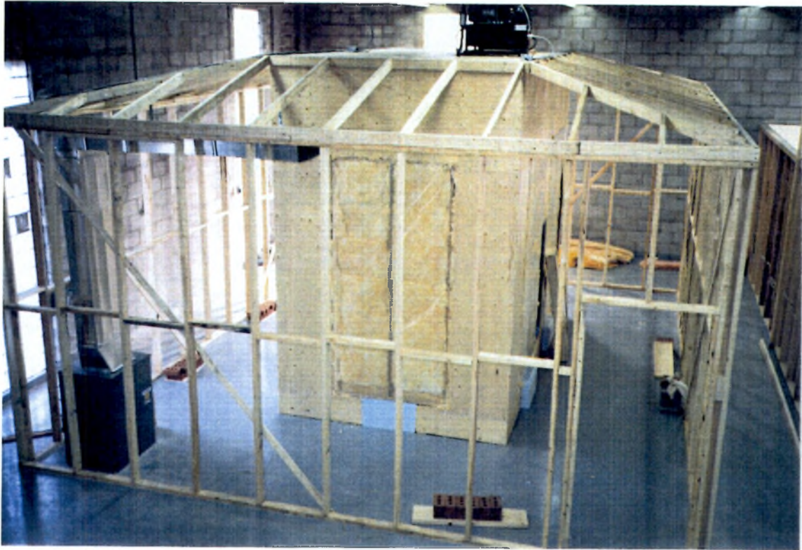
Photo 1 View of test chamber and tent under construction.
