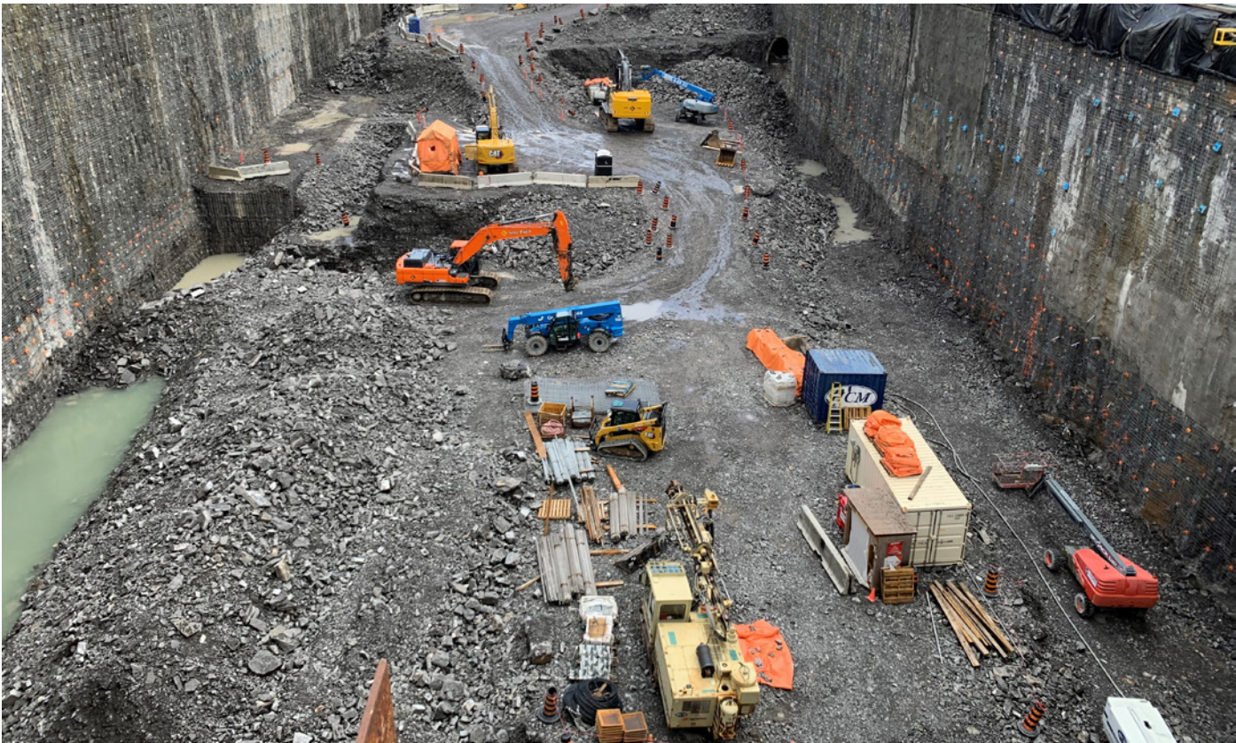
Excavation Work at Parliamentary Precinct
