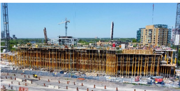
Ādisōke construction site
